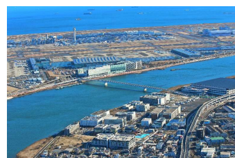
Tamagawa Sky Bridge
